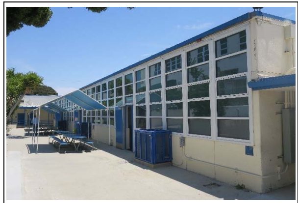
Building E, north façade, view east (ARG, 2021)
