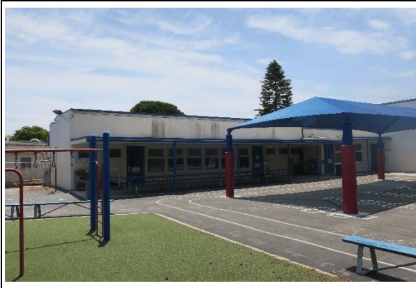
Building G, north façade, view southwest (ARG, 2021)
