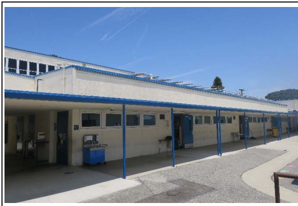
Building E, south façade, view northeast (ARG, 2021)
