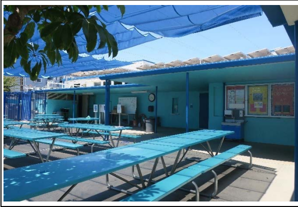
Building A, south façade, view northwest (ARG, 2021)
