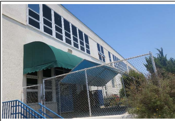
Building B, south façade, view north (ARG, 2021)
