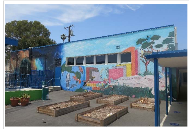
Building C, south façade, view northwest (ARG, 2021)
