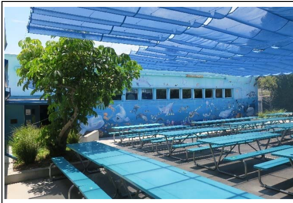
Building C, north façade, view southwest (ARG, 2021)
