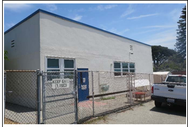
Building G, west façade, view east (ARG, 2021)
