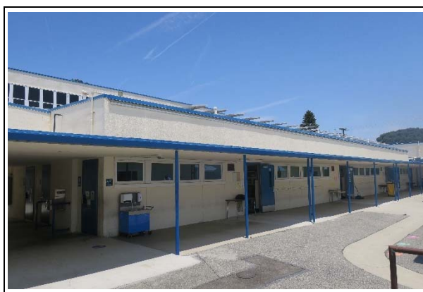
Building E, south façade, view northeast (ARG, 2021)
