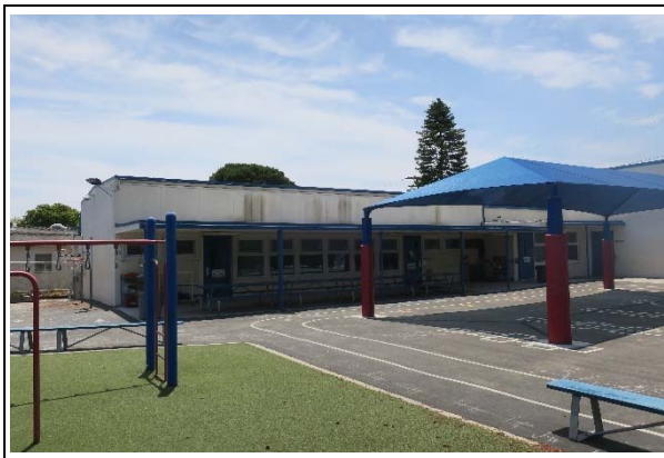
Building G, north façade, view southwest (ARG, 2021)
