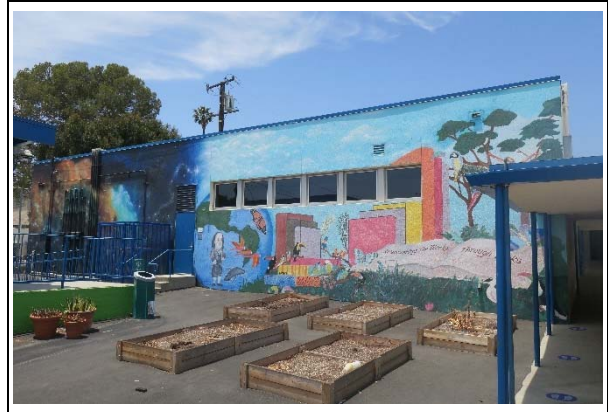
Building C, south façade, view northwest (ARG, 2021)
