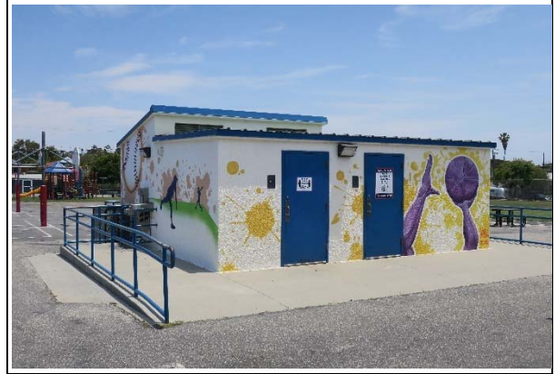
Restroom structure at south end of campus, view southeast (ARG, 2021)
