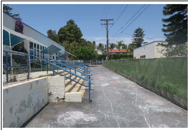
Patios and asphalt paving at east end of campus, view north (ARG, 2021)
