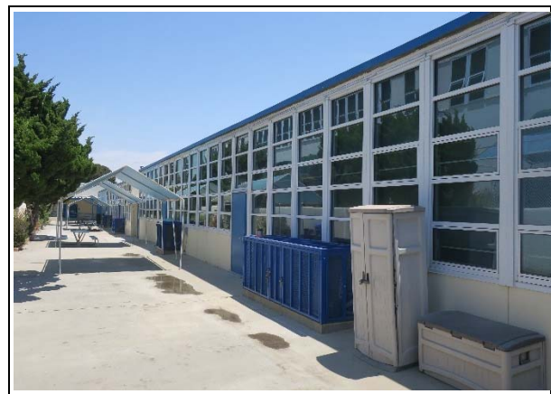
Building D, north façade, view east (ARG, 2021)
