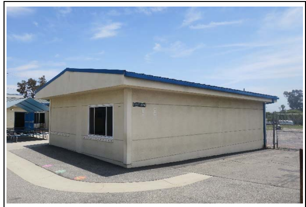
Modular structure, view southeast (ARG, 2021)
