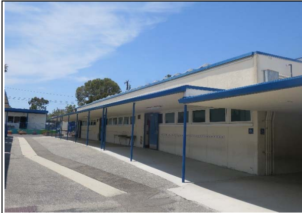
Building D, south façade, view northwest (ARG, 2021)
