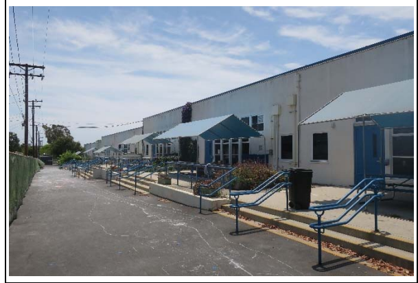
Building F, east façade, view south (ARG, 2021)
