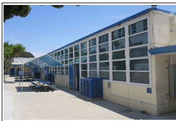
Building E, north façade, view east (ARG, 2021)
