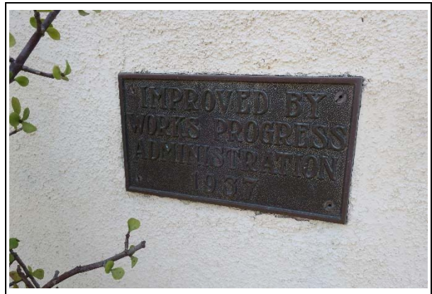
Building B, detail of WPA plaque on north façade (ARG, 2021)
