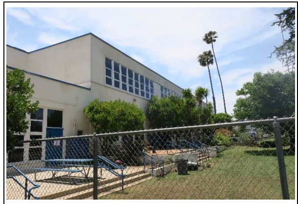
Building B, north façade, view west (ARG, 2021)
