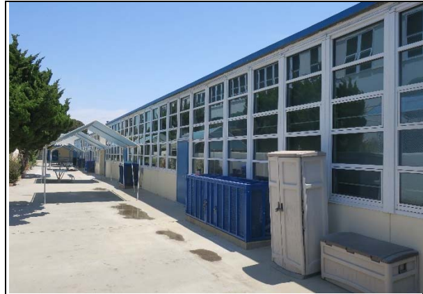
Building D, north façade, view east (ARG, 2021)
