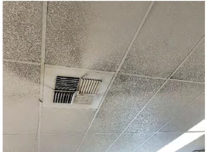
Photo #24: Classroom 75 – ceiling staining observed near HVAC supply registers
