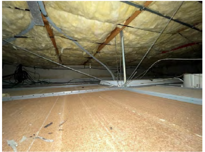
Photo #8: Classroom 71 – light debris in ceiling cavity
