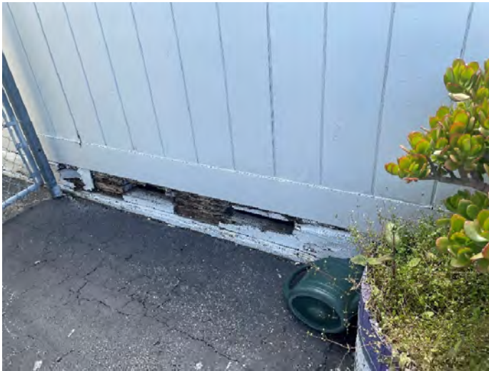
Photo #27: Wood rot observed at the exterior of the bungalows
