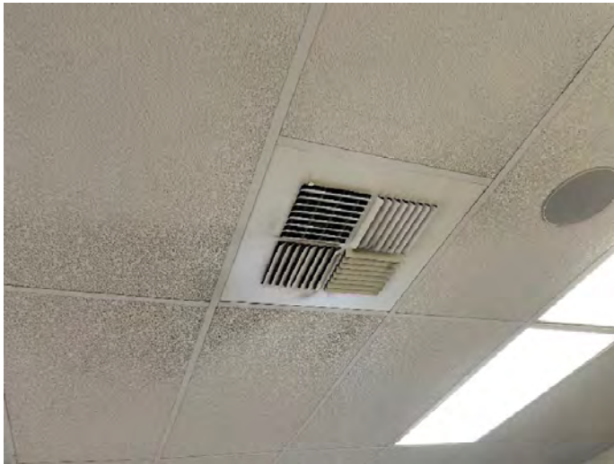
Photo #19: Classroom 74 – ceiling staining observed near HVAC supply registers
