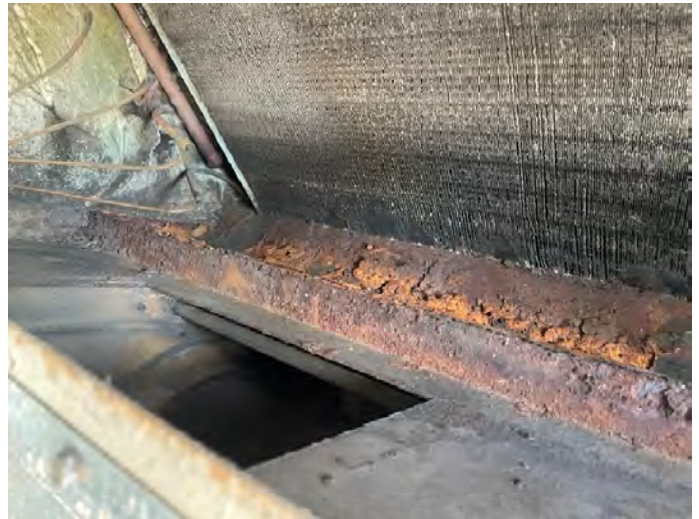
Photo #28: Classroom 71 air handling unit, heavy dust deposition and rusting observed
