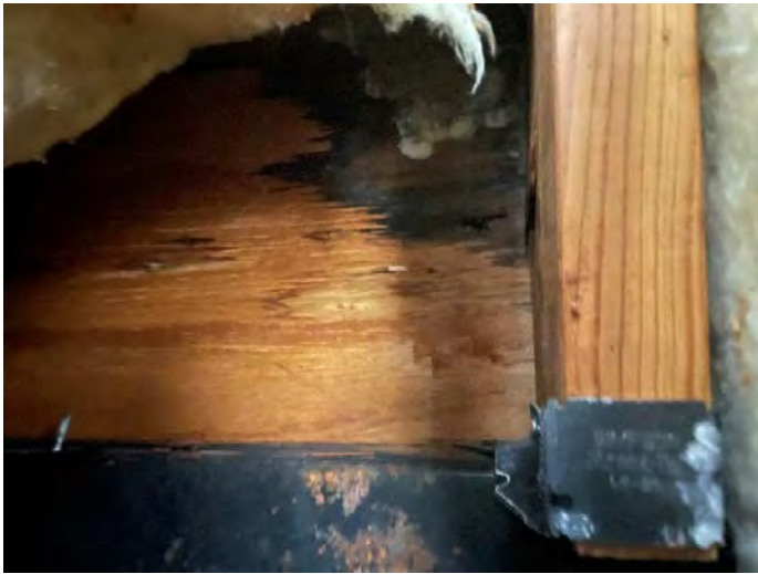
Photo #5: Classroom 70 black staining on wood in ceiling cavity
