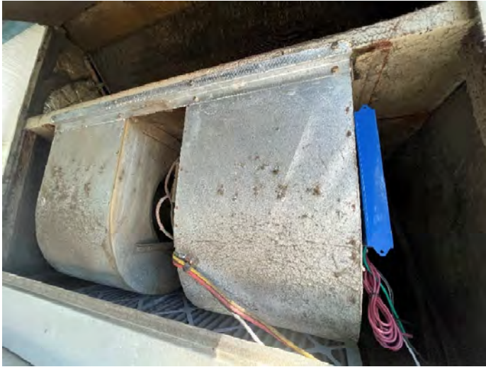
Photo #29: Classroom 71 air handling unit, heavy dust deposition and rusting observed
