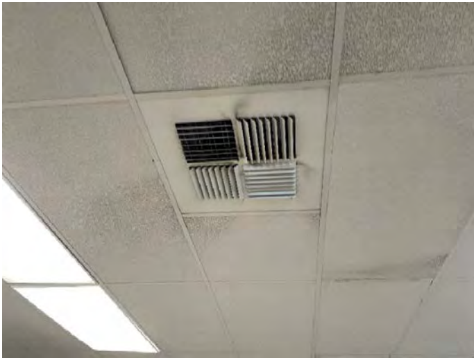
Photo #15: Classroom 73 – ceiling staining observed near HVAC supply registers
