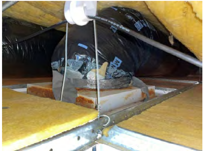
Photo #16: Classroom 73 - rusted HVAC supply
