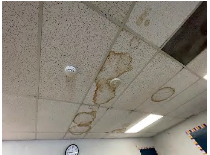
Photo #4: Classroom 70 – water staining on ceiling tile throughout
