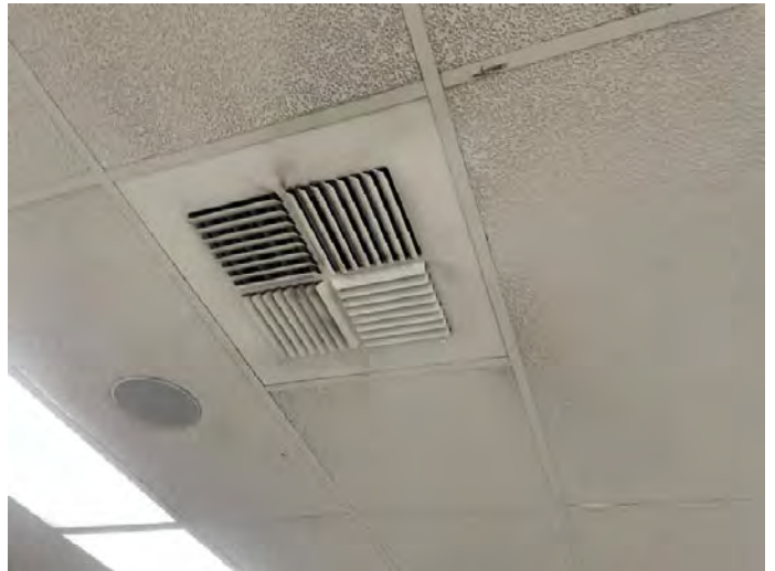
Photo #20: Classroom 74 – ceiling staining observed near HVAC supply registers
