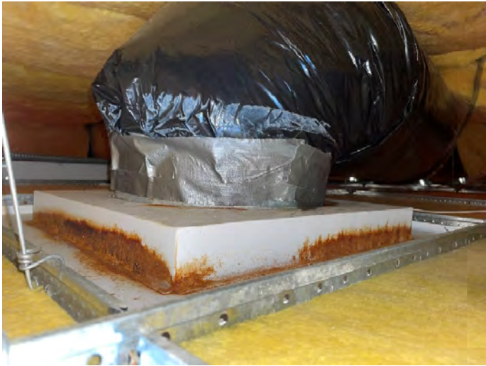
Photo #21: Classroom 74 - rusted HVAC supply
