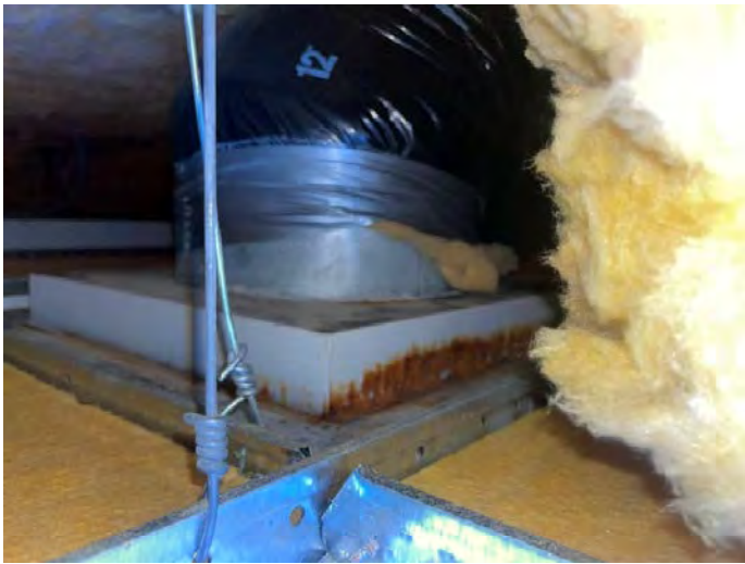
Photo #25: Classroom 75 - rusted HVAC supply
