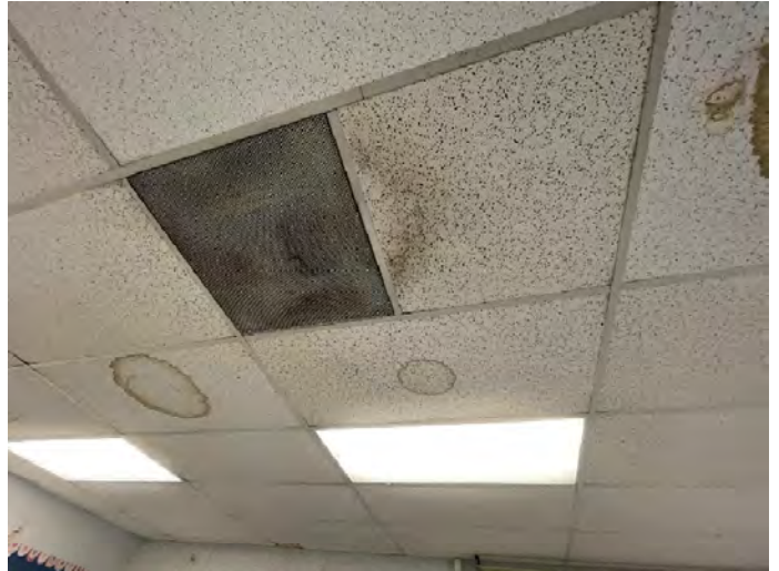
Photo #2: Classroom 70 – water staining on ceiling tiles throughout
