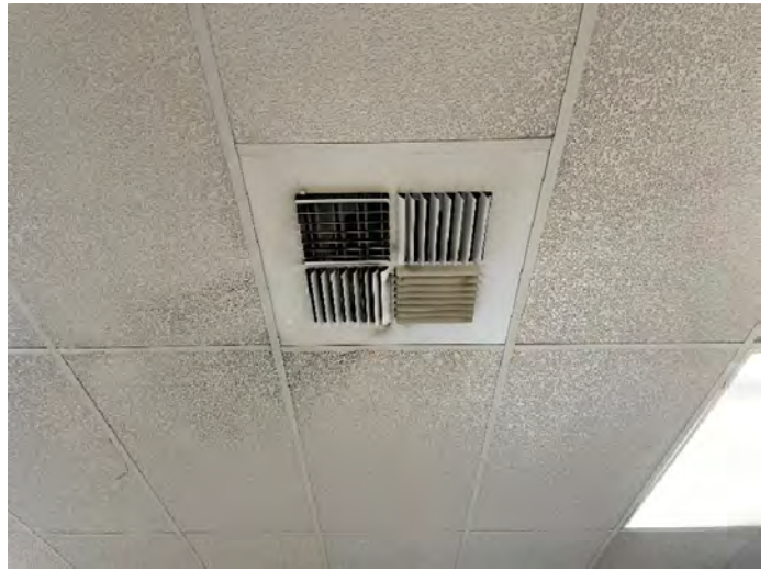
Photo #14: Classroom 73 – ceiling staining observed near HVAC supply registers
