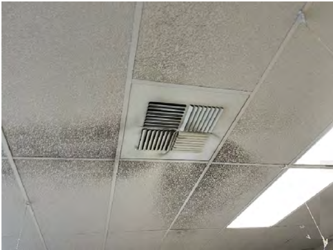
Photo #23: Classroom 75 – ceiling staining observed near HVAC supply registers
