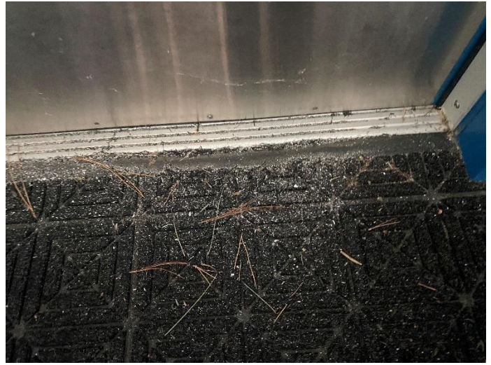
Photo #6: Bldg C, Classroom 13 – visible smoke related particulate on flooring at door entry
