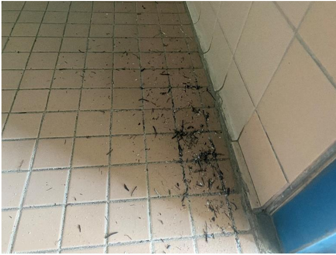
Photo #5: Bldg H, Restroom – Heavy fire smoke debris on flooring throughout room
