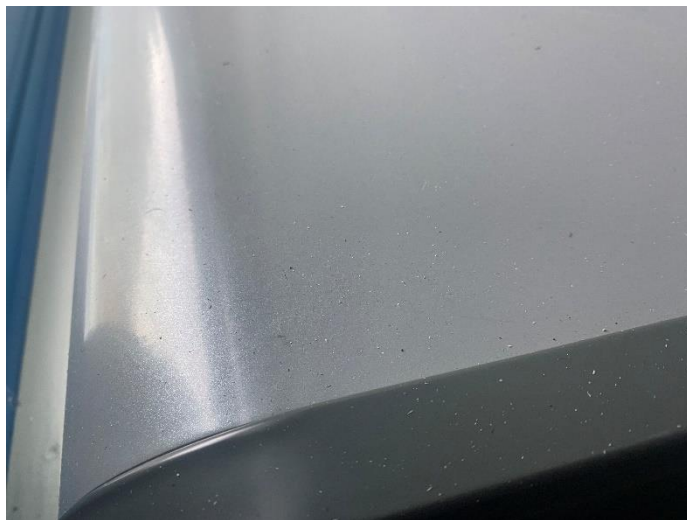
Photo #2: Smoke and fire debris identified on exterior surfaces
