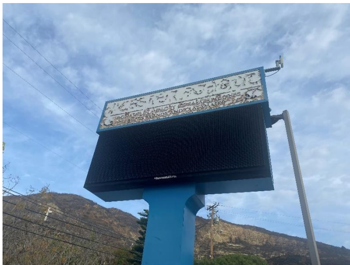
Photo #1: Heat damage of school sign
