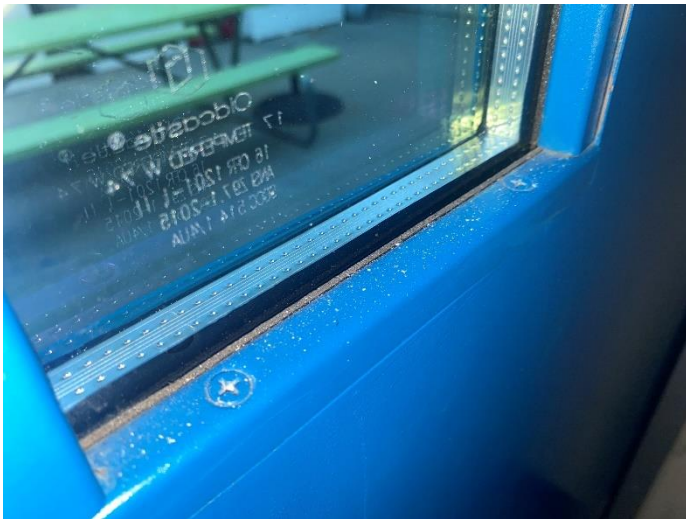
Photo #7: Bldg F, Classroom 2 - visible smoke related particulate on interior door
