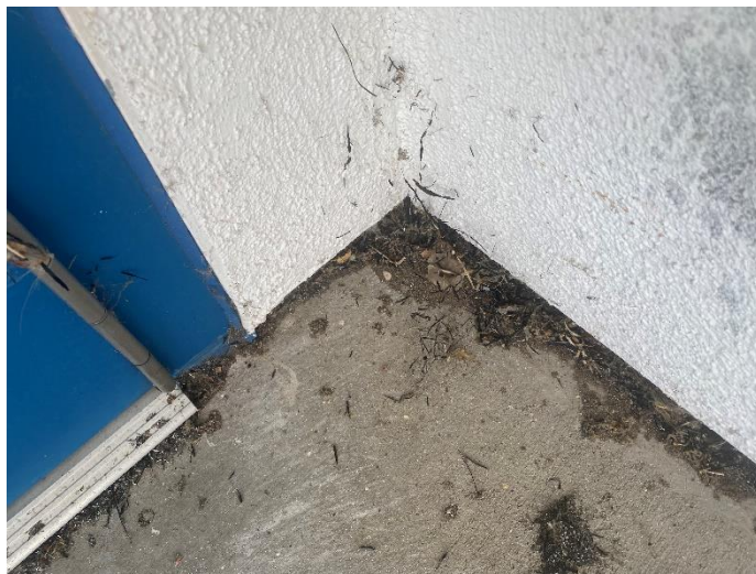
Photo #2: Smoke and fire debris identified on exterior surfaces
