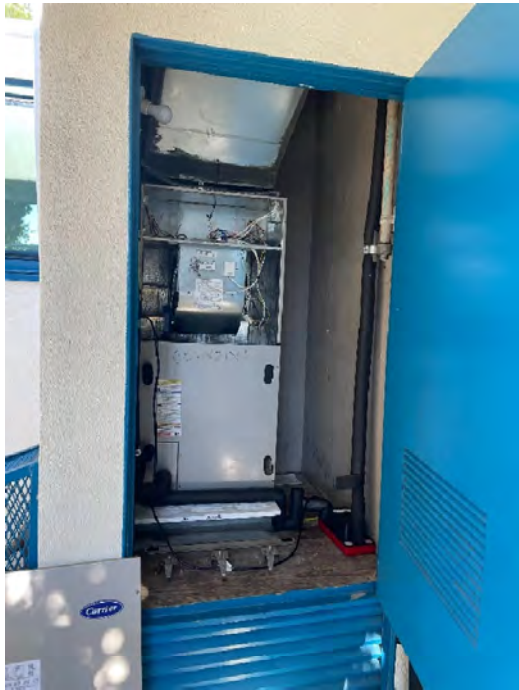
Photo #13: HVAC AHU (representative/example) – Building C, Rm 13
