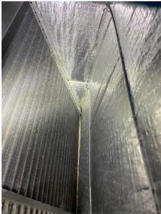
Photo #15: HVAC AHU (representative/example) – Building C, Rm 13 – surfaces clean
