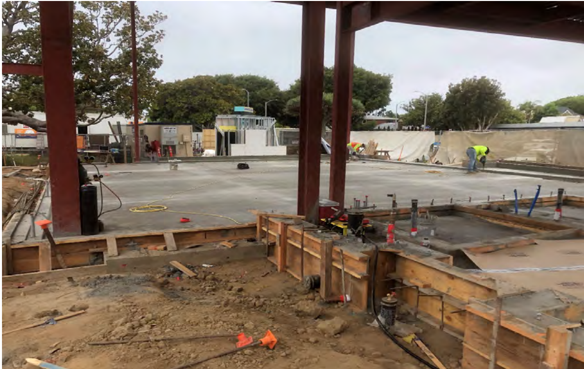
The slab on grade at the rehearsal building has been poured.
