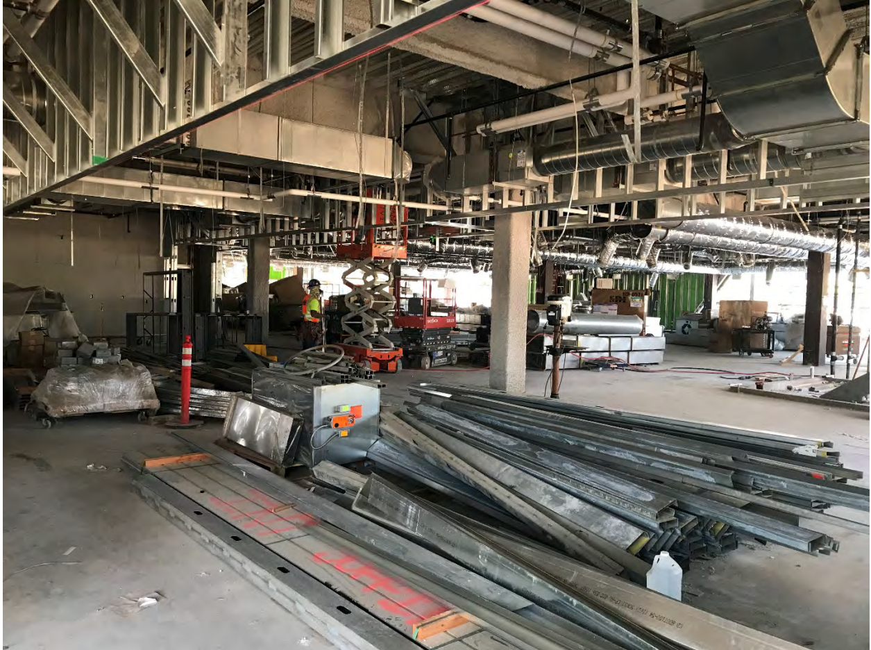
This view shows how complex the work is on the cafeteria and its overhead utilities.
