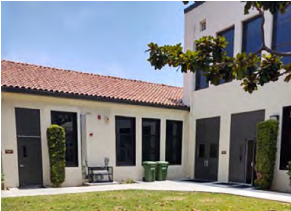
New windows on the administration area of the main building.
