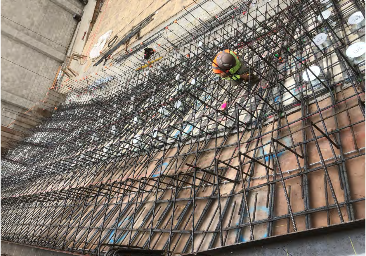
Rebar being installed at the upper seating area.
