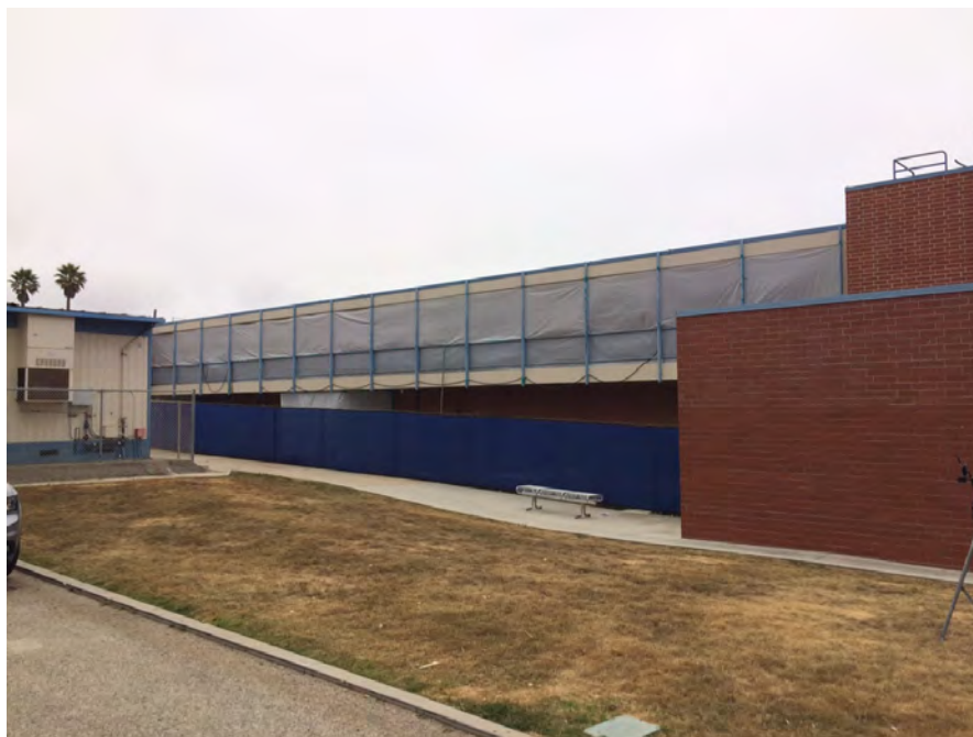
The former junior high building, sealed during abatement work.
