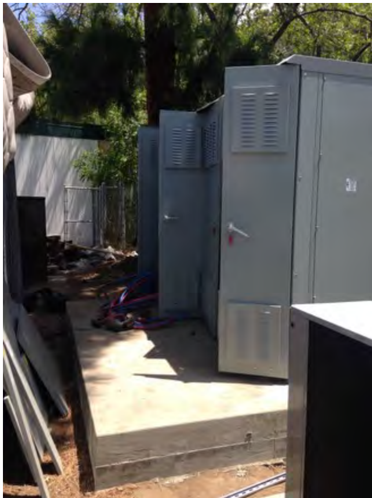
New electrical switchgear awaits power-up.
