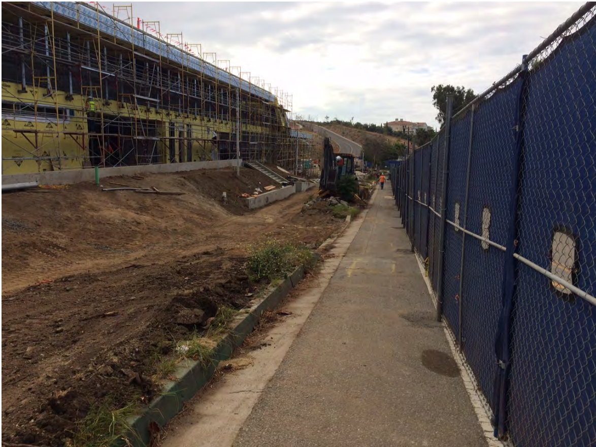
On the Morning View Drive side of the building, existing curbing and sidewalks are being removed.
