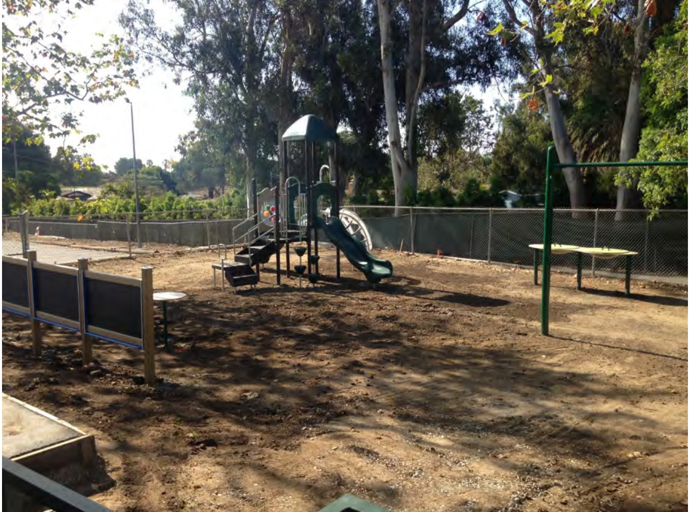
The upper play area in progress.
