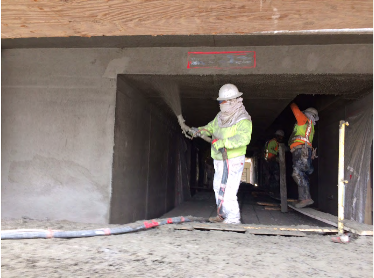
Coating a breezeway on the north side of the building.
