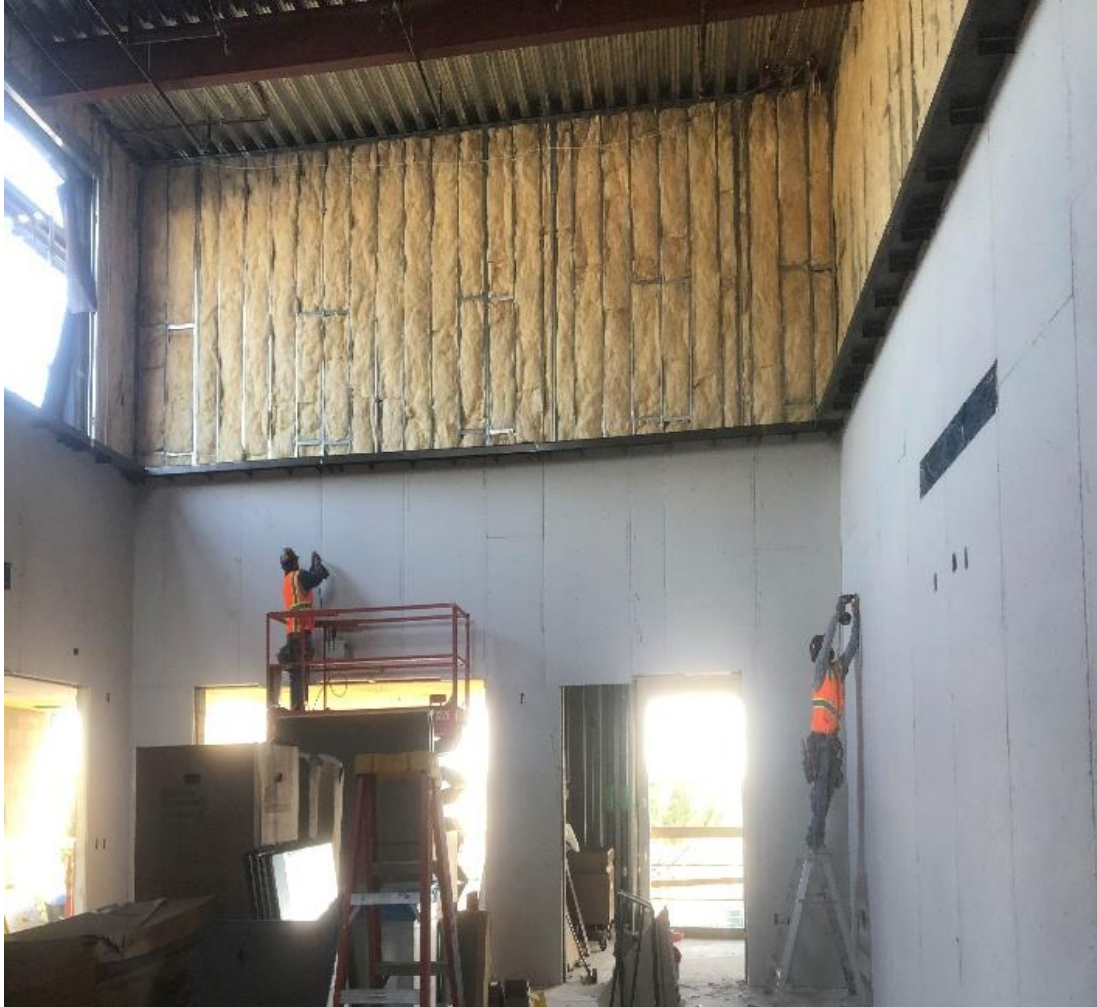
Contractors work on the interior of the choir room.
