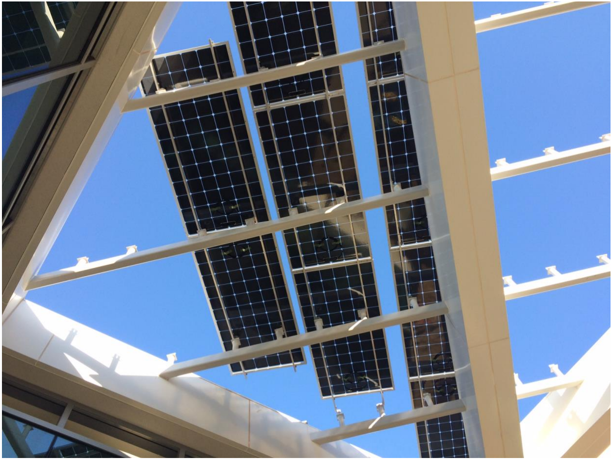
The building's solar panels as seen from below.
