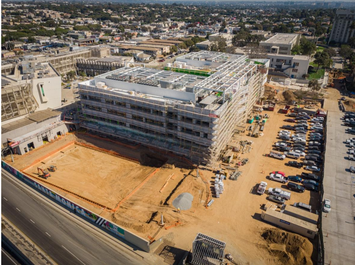
The site as seen from the north. The area surrounded by orange fencing in the foreground will eventually become the pool.
