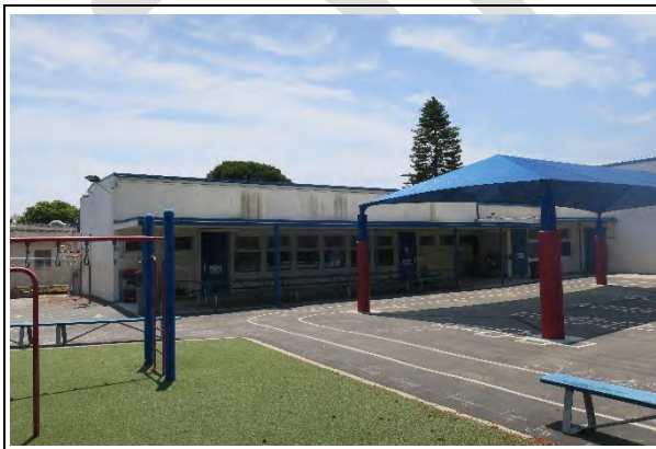
Building G, north façade, view southwest (ARG, 2021)
