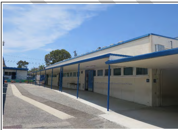
Building D, south façade, view northwest (ARG, 2021)
