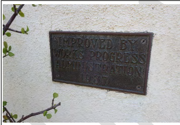
Building B, detail of Works Progress Administration Plaque on primary (north) façade (ARG, 2021)
