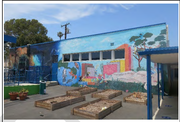
Building C, south façade, view northwest (ARG, 2021)
