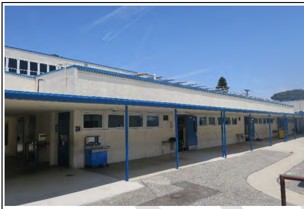
Building E, south façade, view northeast (ARG, 2021)
