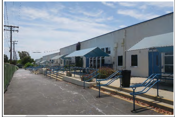
Building F, east façade, view south (ARG, 2021)
