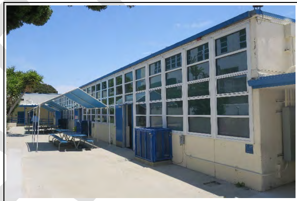
Building E, north façade, view east (ARG, 2021)
