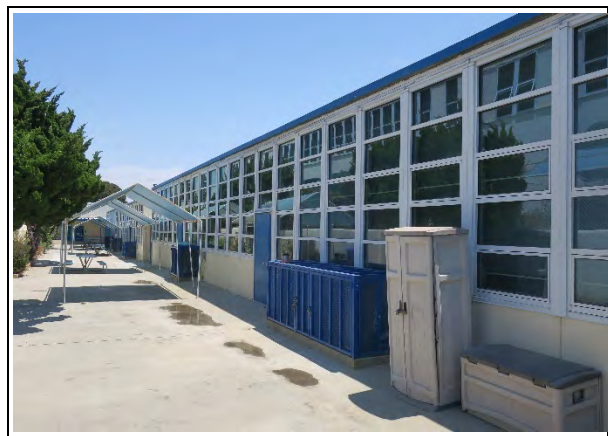
Building D, north façade, view east (ARG, 2021)
