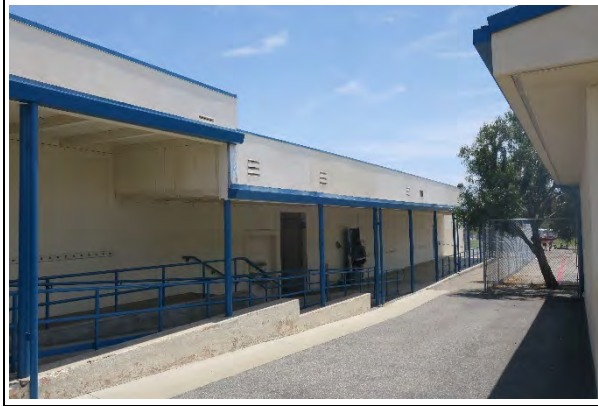
Building F, west façade, view southeast (ARG, 2021)
