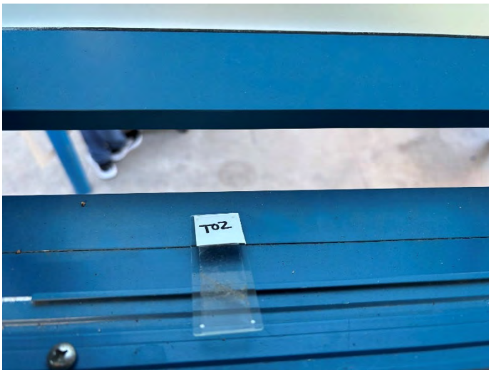
Photo #7: Building C – Girls Restroom – Windowsill – T-02
