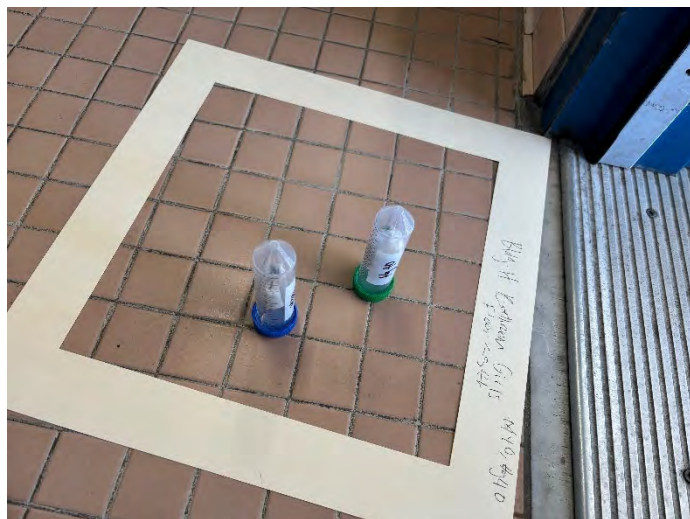
Photo #79: Building H – Girls restroom – Floor – M/Hg-40
