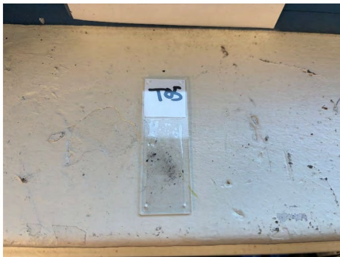
Photo #50: Building E – Room 7 – Windowsill – T-05
