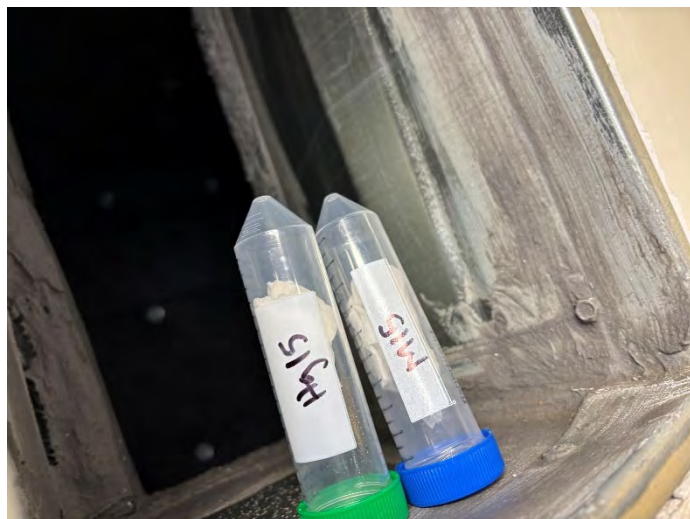
Photo #31: Building A – Room 20 – HVAC Supply – M/Hg-15
